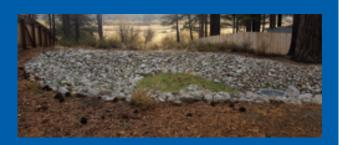
**Infiltration basins** are shallow, man-made ponds or engineered wetlands that allow stormwater to infiltrate into the soil. Some basins can also include dry wells or other overflow systems to prevent flooding.
