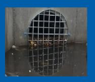
**Pipe grates** are placed over a pipe to catch solid materials traveling through the pipe.
