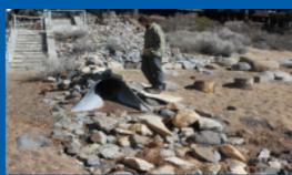
**Rip-rap** is loose stone used to prevent erosion by slowing down fast moving water.
