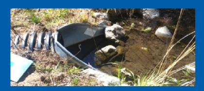
**Culverts** are tunnels that carry an open drain under a road.
