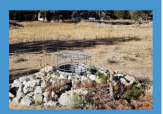
**Dry wells** are structures that allow water to percolate directly into the ground, as well as direct any excess water further downstream into other stormdrains, basins, and sediment traps. They may look like raised stormdrains and can be found along your neighborhood streets. Some dry wells are used as overflows within basins to collect and direct excess water out of the basin to prevent flooding in roads and neighborhoods..
