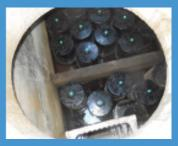
**Sediment traps (or vaults)** are underground structures that allow sediment to settle out of flowing stormwater and remain in the bottom of the trap, which can be emptied when full. Water escapes via a pipe, but only when the trap is full. In some versions of this system, the traps are large enough that water cannot escape via a pipe; instead, water infiltrates into the ground or evaporates.
